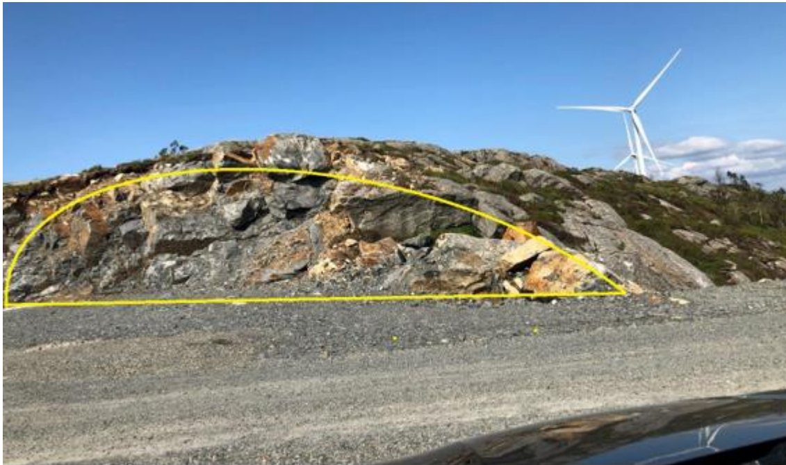
Backfill with local material and soil
