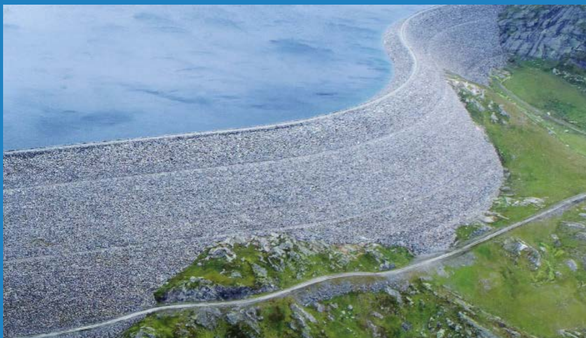
Storvassfyllingsdam (foto: Statkraft Energi AS):
