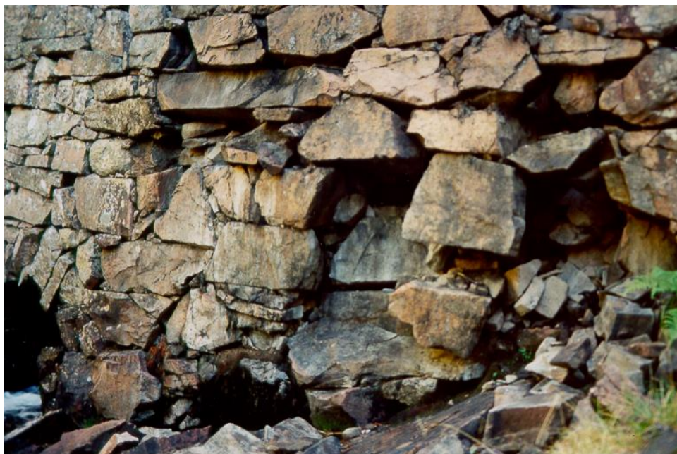
> Figur 8-2. Utrast stein i damtå under utbuling.
